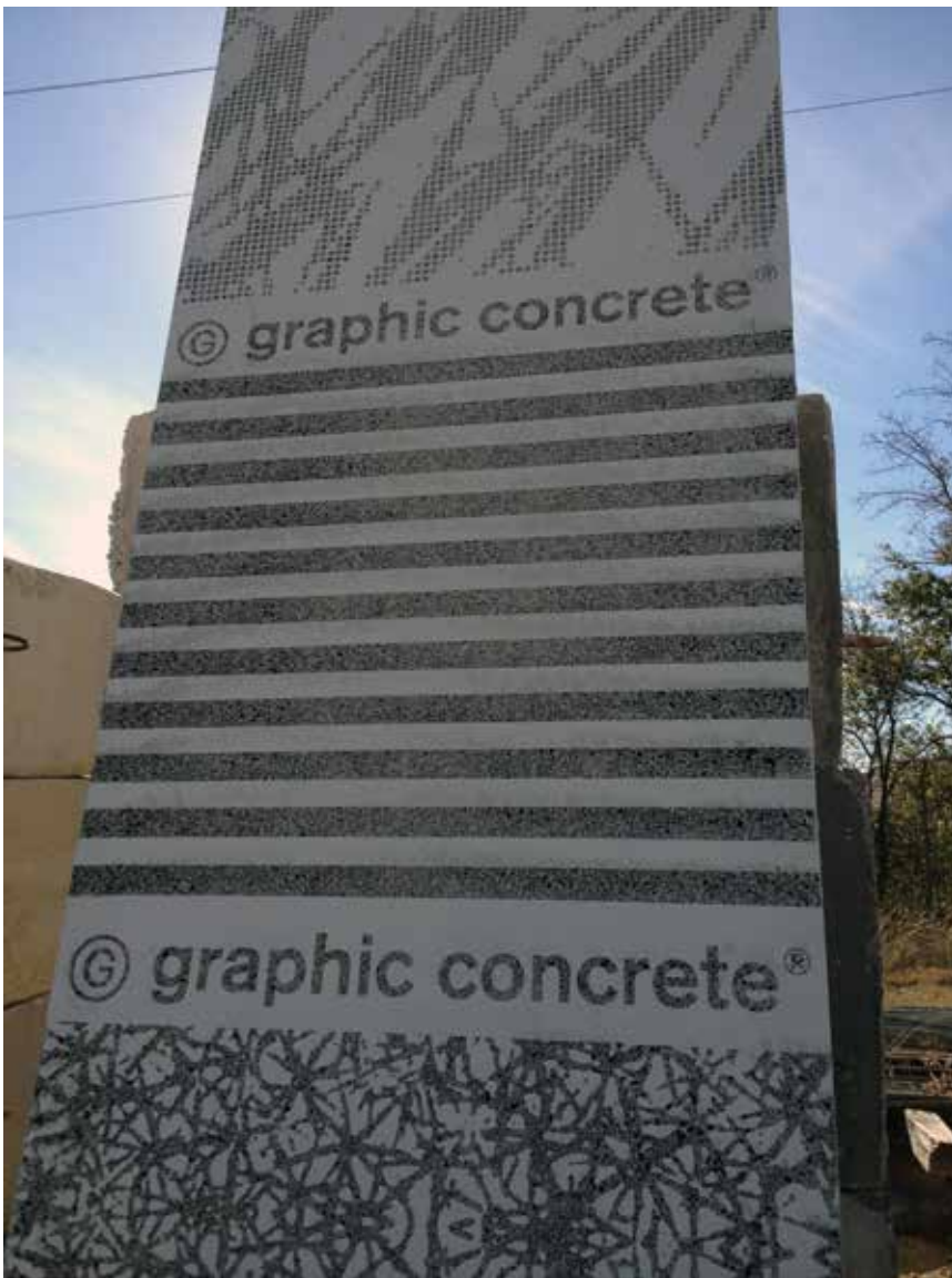
This photographic reproduction was created using a CNC router on a panel with white cement and black aggregate. Photo: Gate Precast.
