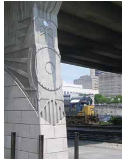
Bridge designers are incorporating formliner designs into their structures, especially in highly visible locations. This design on a bridge in Nashville ties into the railroad yard that the bridge spans. Photo: Scott System.
