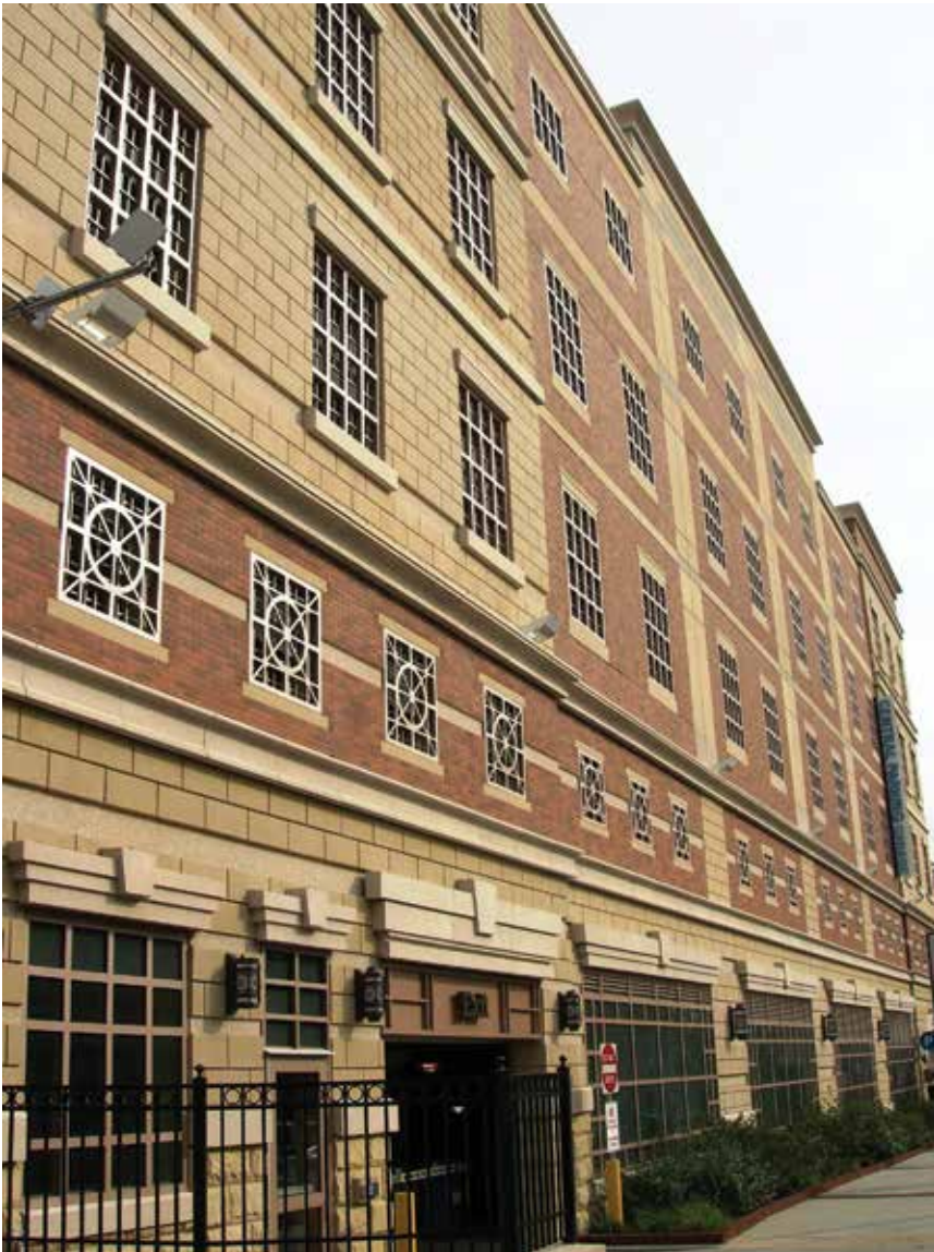
Architects are becoming more creative in combining textures, shapes, and designs to create distinct aesthetic treatments in precast concrete panels. These panels with embedded thin brick using Scott Brick Snap Systems are featured on the parking structure for Lancaster Newspaper in Lancaster, Pa. Photo: A.L. Patterson.
